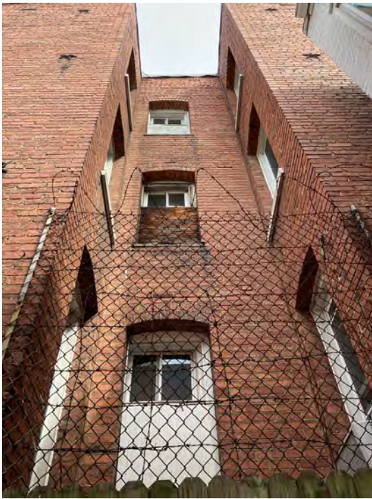
LIGHT WELL AT 747 10 TH SE
