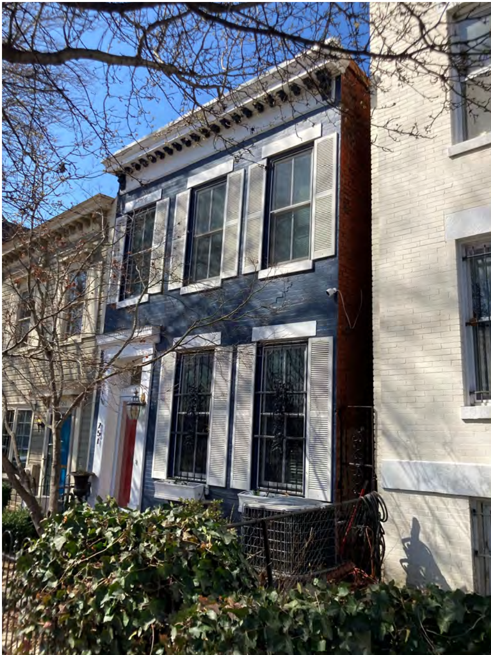
EXISTING FRONT FACADE
