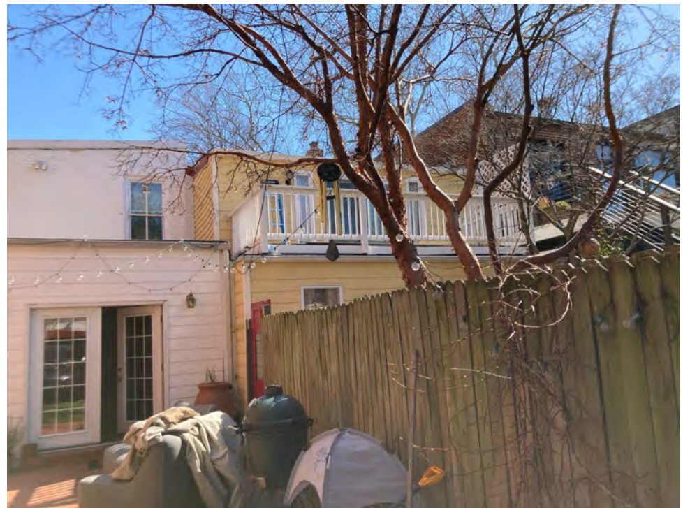
REAR FAÇADE, LOOKING SOUTH
