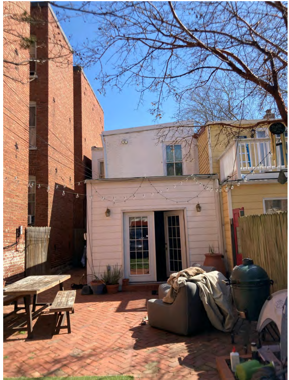
EXISTING REAR FACADE
